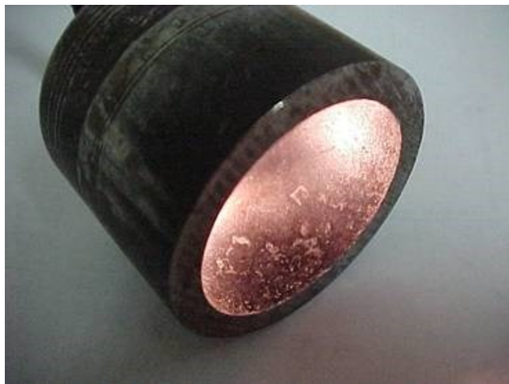
Before applying ELC
